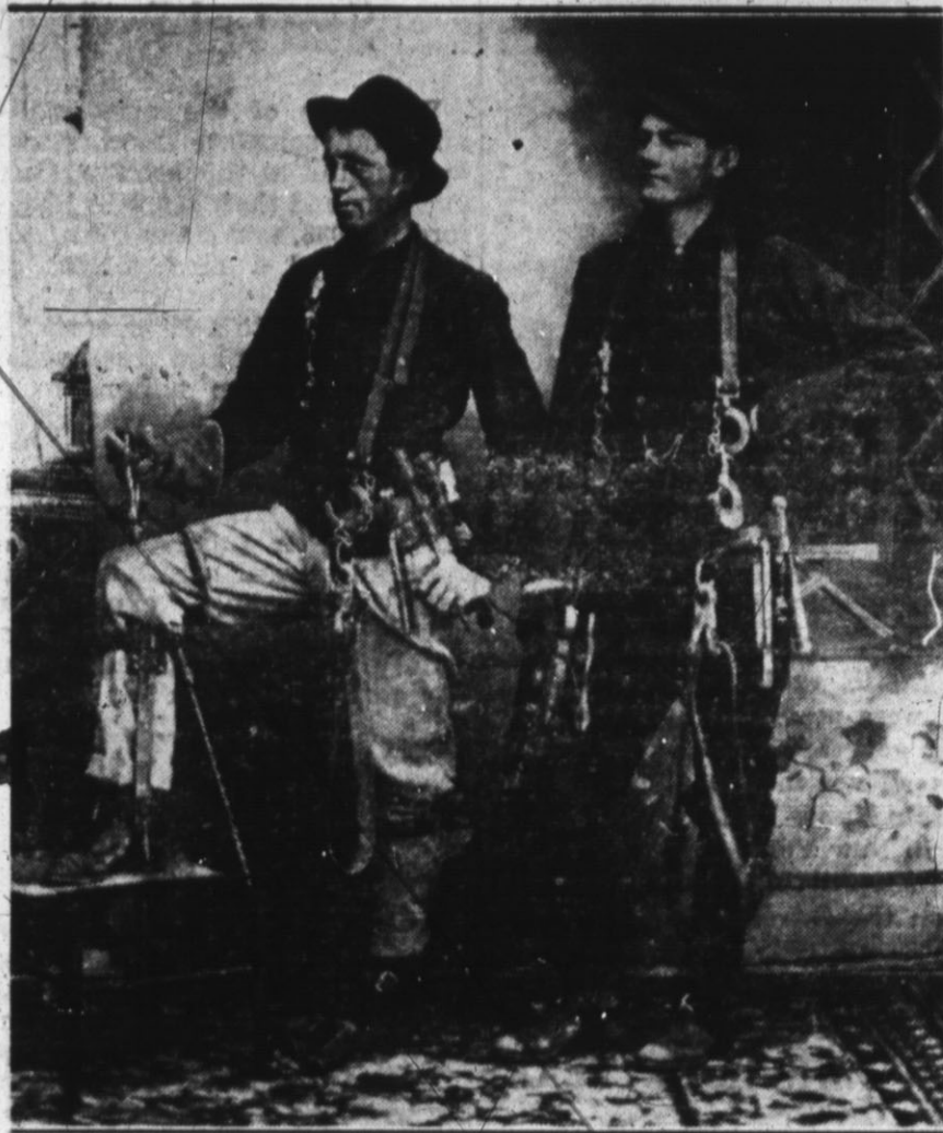
Tom Hindman, right, and Press Dyer are shown in the above picture after a hard day's work on telephone lines. The picture was made in 1908; many old timers will remember when these two young men were kept busy with line repairs.
