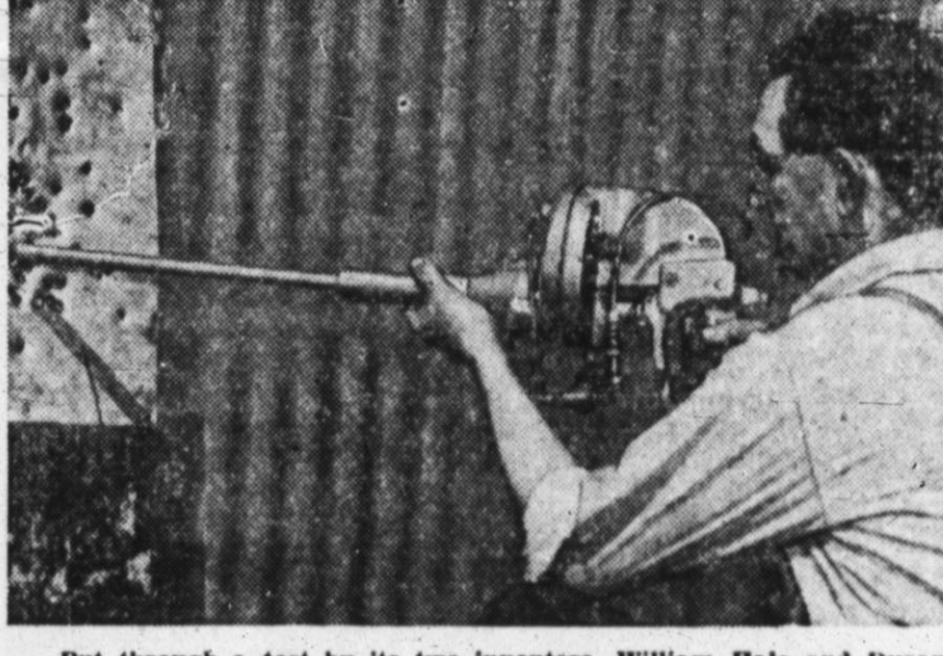
Put through a test by its two inventors, William Hale and Durand Beam, this rifle fired 10,000 shots per minute—with absolutely no noise. The rifle operates with compressed air. It reduced three-inch oak planks to kindling and turned airplane armor plate into steel mosquito netting. It resembles a sub-machine gun, and when it starts firing the barrel gets cooler instead of heating up.
