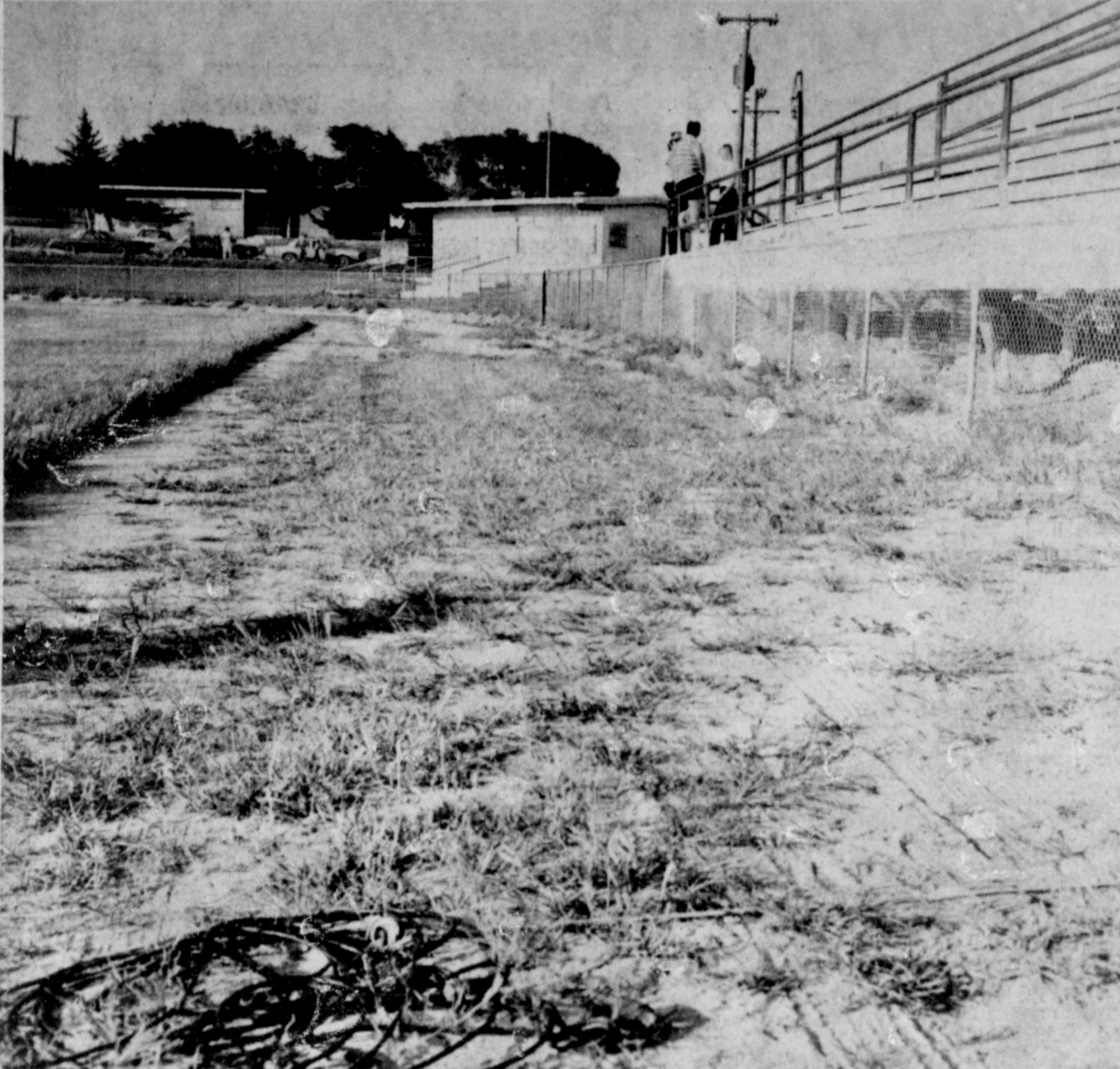
THIS IS WHY MULESHOE NEEDS A NEW TRACK --This picture graphically illustrates one of the reasons a new all-weather track is needed at the MHS football field. These clumps of grass, weeds and sand burrs have filled the track, creating hazards for all runners. An effort will begin in the very near future to try to collect enough funds to install an all-weather track and rebuild the west side stands into the 'home stands' for Benny Douglass Stadium.
