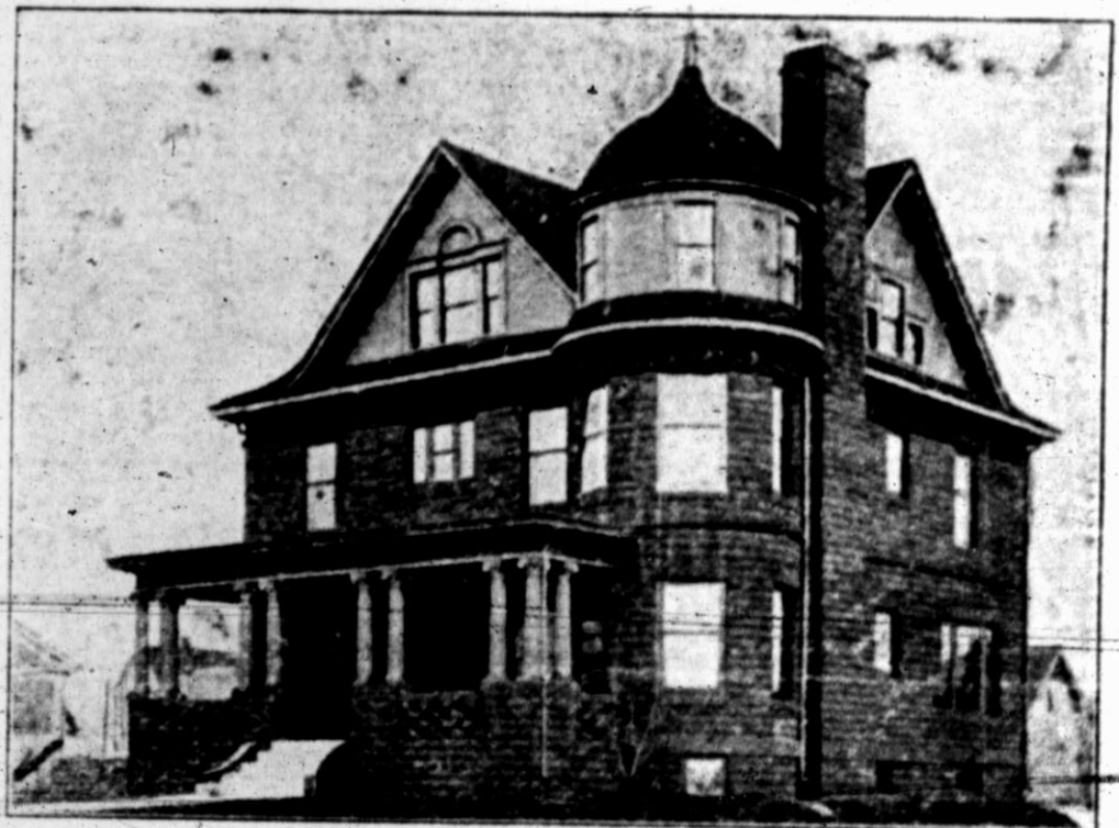
See J. L. Johnson for Waterproof Building Blocks. Also for a Turn Key Job. Factory, Hereford, Texas. Phone 324.
