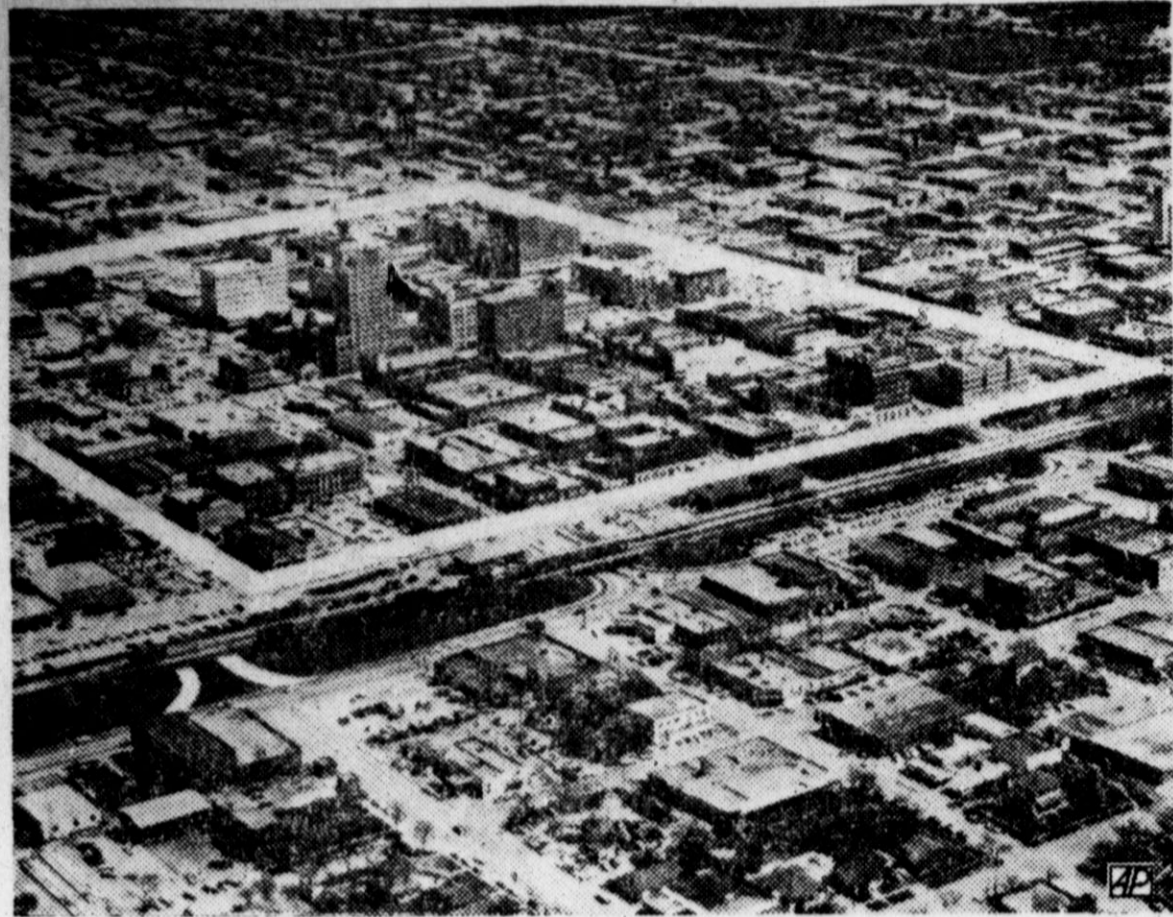
WHOLESALE ATTACK ON "DOWNTOWN BLIGHT"—All streets and sidewalks in this outlined area of downtown Abilene will be torn up and rebuilt in the city's attack on "downtown blight." In left foreground is site of third underpass which will help unite business districts on opposite sides of railroad. (AP Wirephoto)
