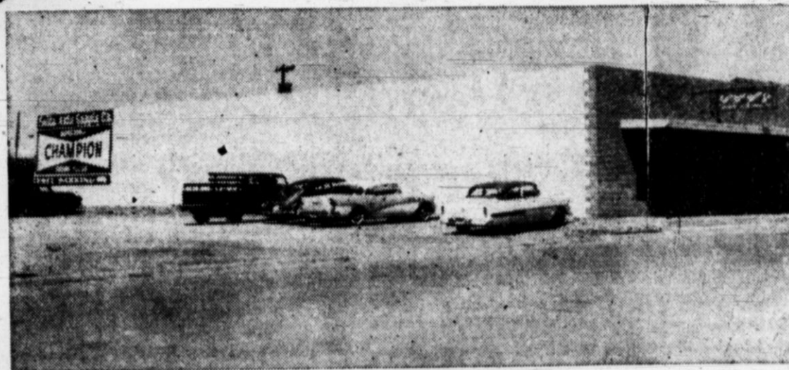
Our Big New Modern Building at 115 Schley with Plenty
