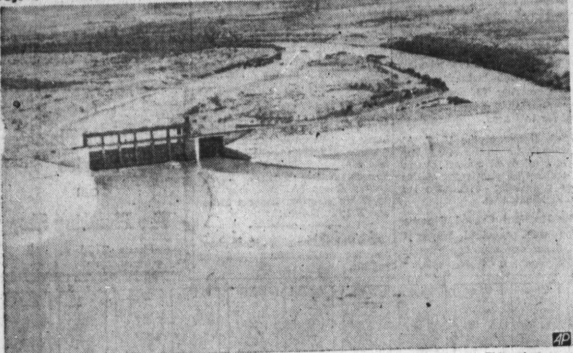
DRY LAND IN FALCON RESERVOIR—This aerial view of Falcon Dam and reservoir shows the low level of water in the lake. The ground in the center and much of that to the left is usually covered with water. This photo was taken when the water was at its highest level in weeks after recent rains had raised the level 2 feet. (AP Wirephoto)
