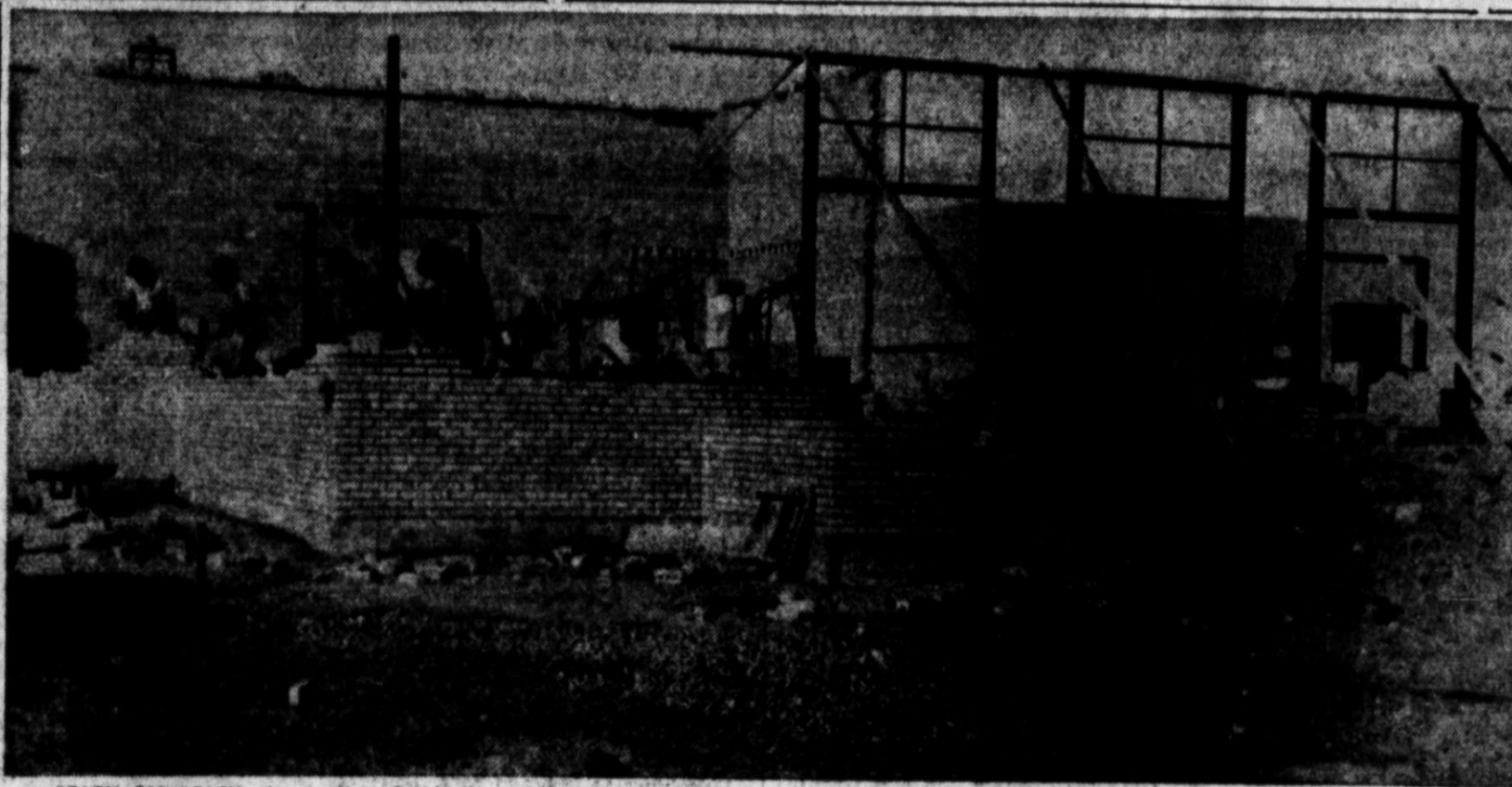
BRICK BY BRICK the walls of the front of the new High School auditorium are going into place, though a delay in the delivery of structural steel has slowed the overall progress of the construction work.
