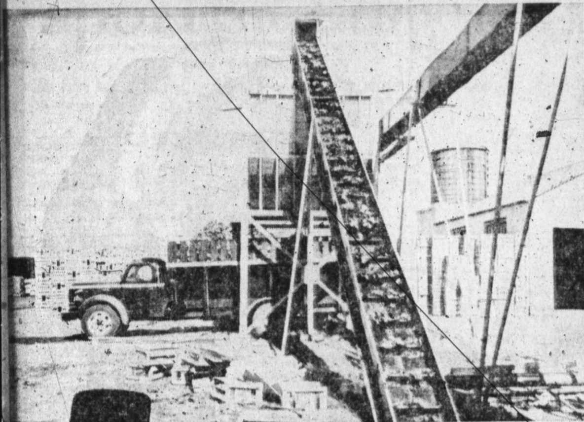
CARRYING OFF THE STRIPPINGS is this elevated conveyor. This is an endless affair that carries off the trimmings from the packing line to waiting trucks. The strippings or waste lettuce is hauled to nearby pastures for cow feed. This picture was made at the Charles Huston Company here Tuesday afternoon. Staff Photo.
