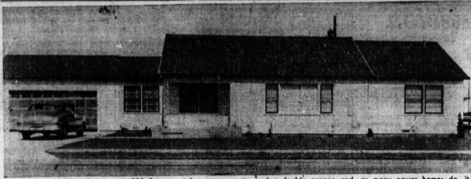
THE ED LOERWALD home at 222 Star street has seven rooms and a double garage and, as many newer homes do, it has double windows all around. Brand Staff Photo.
