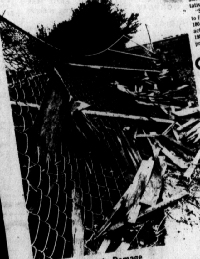
Possible Tornado Damage
