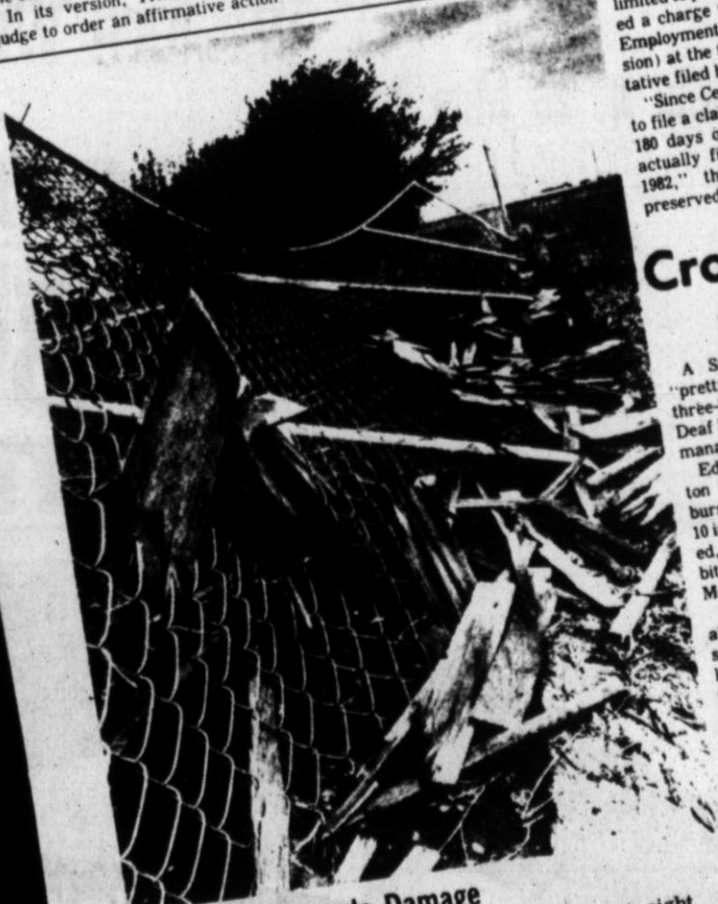
Possible Tornado Damage
