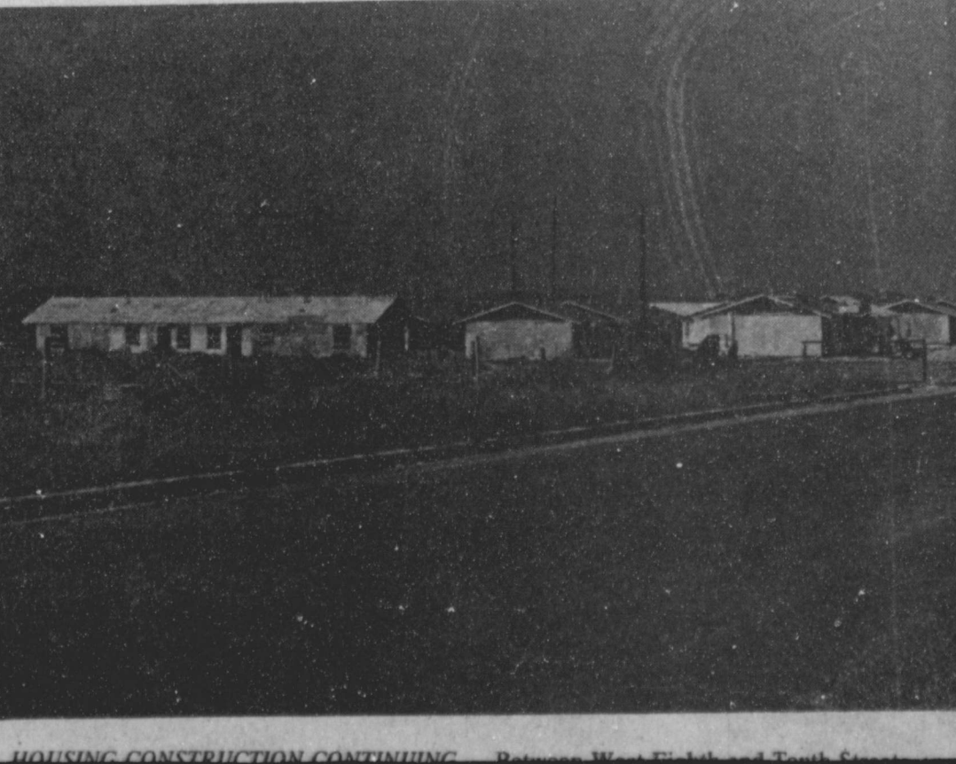
HOUSING CONSTRUCTION CONTINUING
