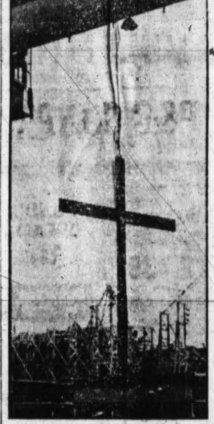
A symbol of peace sways through the air on a journey to war at the Marshfield yards, Sausalito, Calif. An alert pho- tographer snapped the "cross" on its way to becoming part of a ship being built for war duty.
