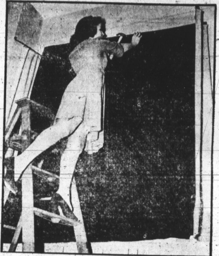
A curtain of felt material provides protection in blackouts. Material is put on a flexible piece of wood with thumb tacks and is hung from the top of the window just like a picture. Not only is light concealed, but felt absorbs splinters in case of shattered glass. Miss Margo Lundgren shows how easily this type of curtain is hung.
