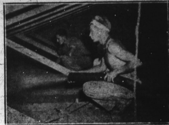
Shows attic of residence with THERMAL WOOL being blown in.
