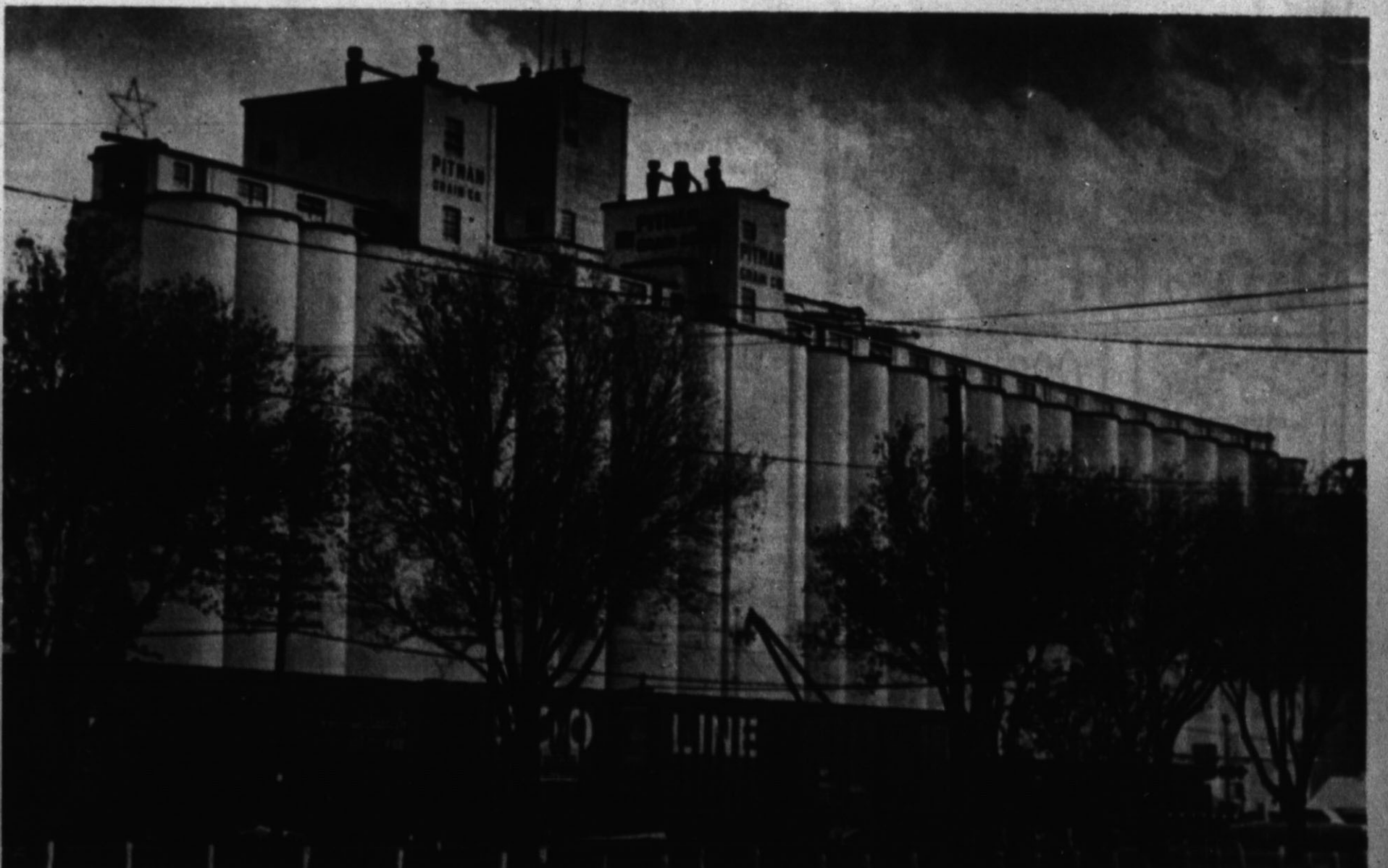
TOWERING HIGH above Hereford is Pitman Grain Company, one of the largest structures erected in Deaf Smith County. The huge complex, located just south of the railroad tracks on South Main St., has a capacity of nearly 3 million bushels of grain. The highest point atop the elevator reaches some 165 feet above the ground and offers a magnificent view of the city. (Hereford Brand Photo)
