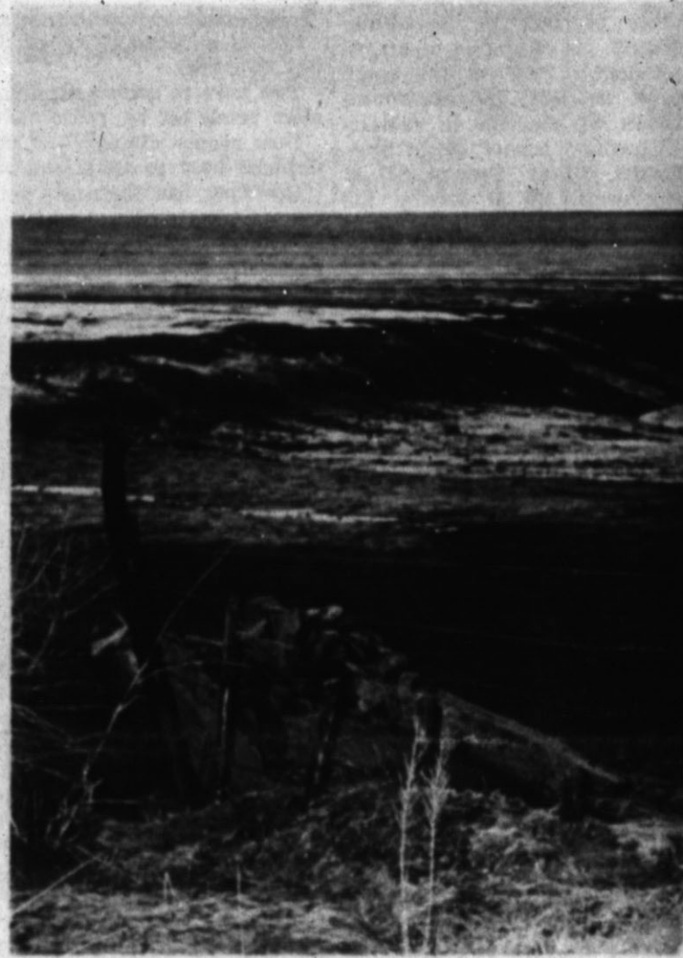
AFTER TORRENTIAL RAINS — Water flows from fields and into a bar ditch approximately 8 miles east of Milo Center following torrential rains in that area Tuesday evening.
