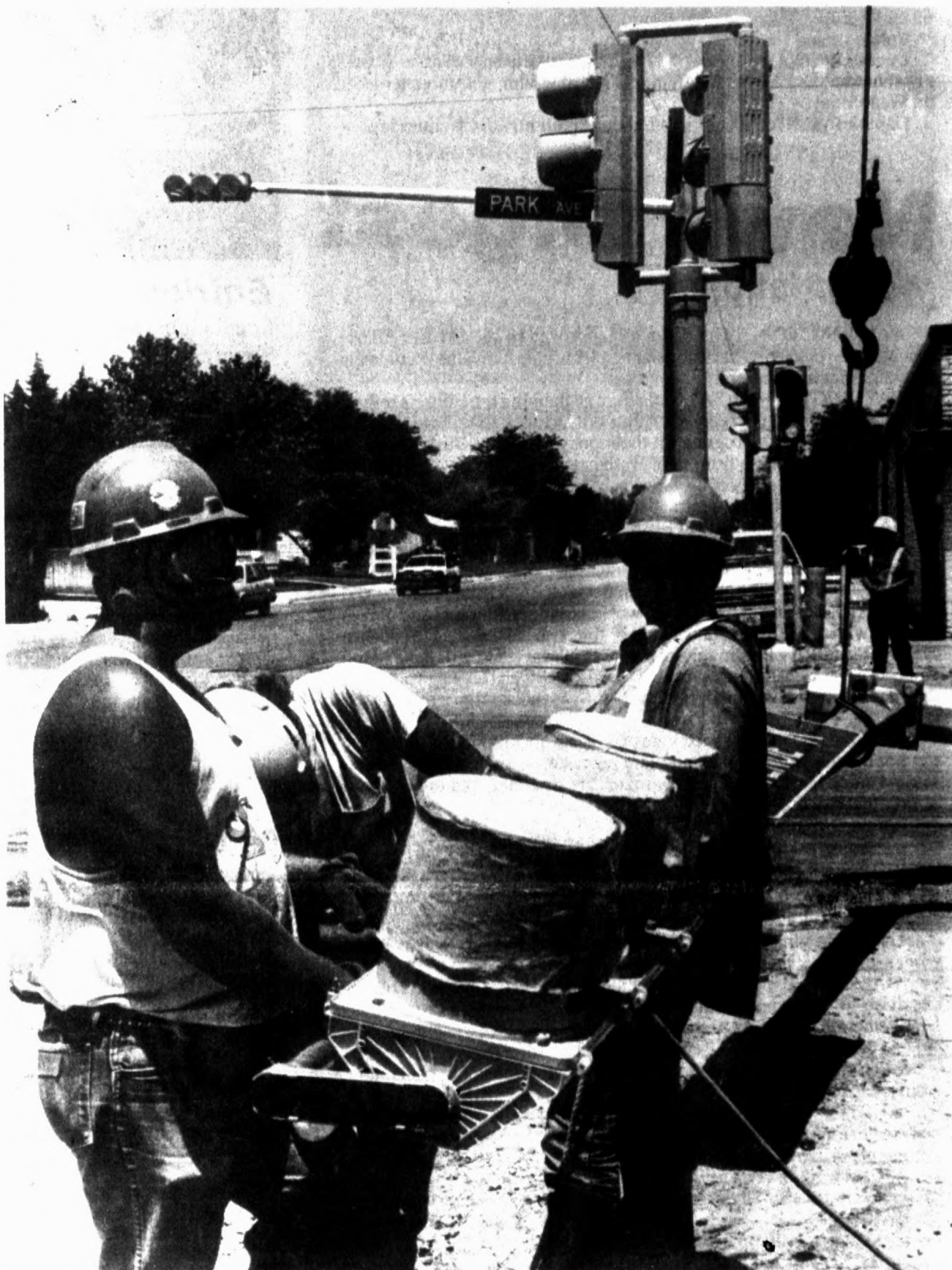
Traffic lights going up
