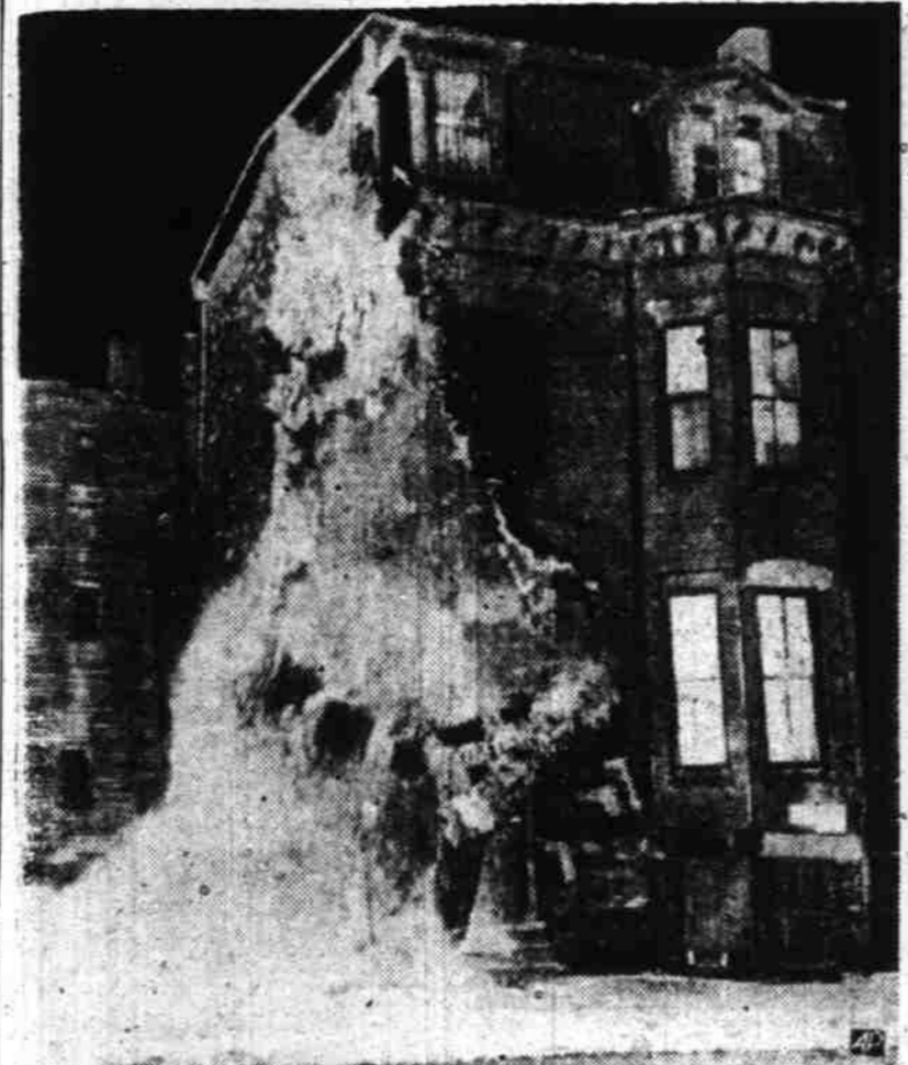
WALL COLLAPSES AT BOSTON—The wall of this three-story brick rooming house collapsed at Boston shortly after police evacuated the occupants. (AP Wirephoto).
