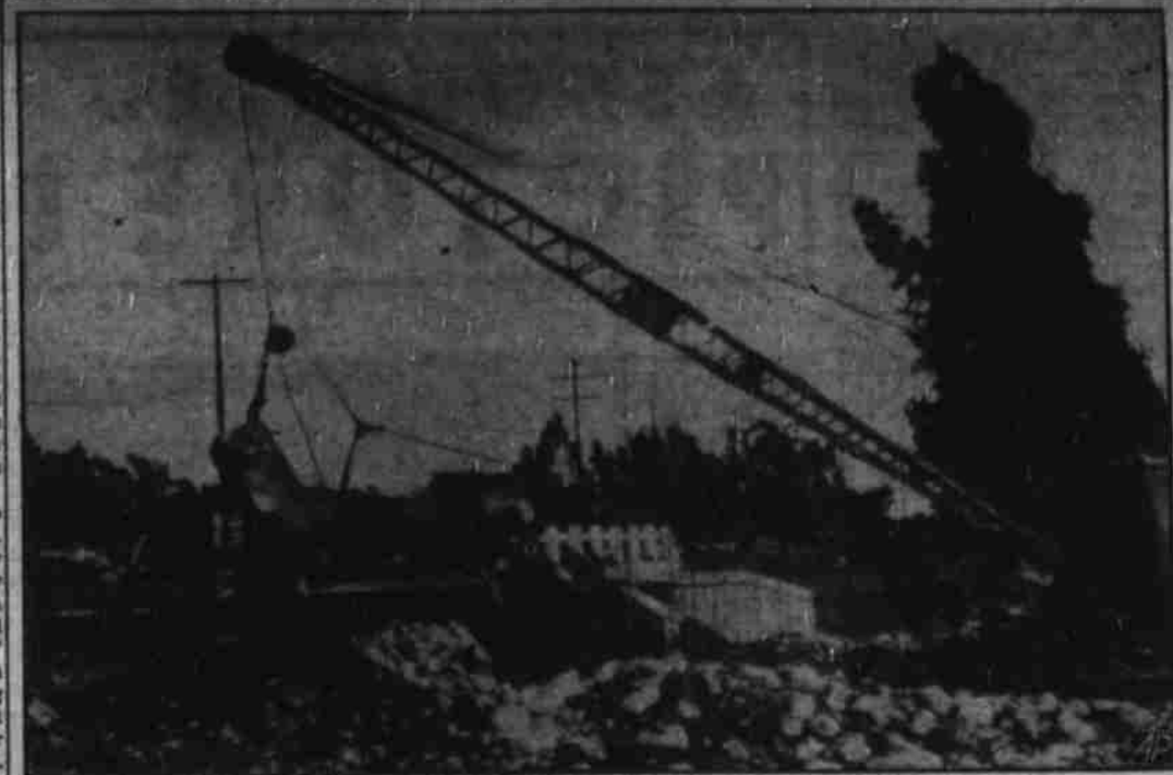
A big shovel is shown in action clearing a boulevard in San Bernardino, Calif., one of the main arteries to Los Angeles. The highway was covered with several feet of gravel in the recent flood, which isolated San Bernardino.
