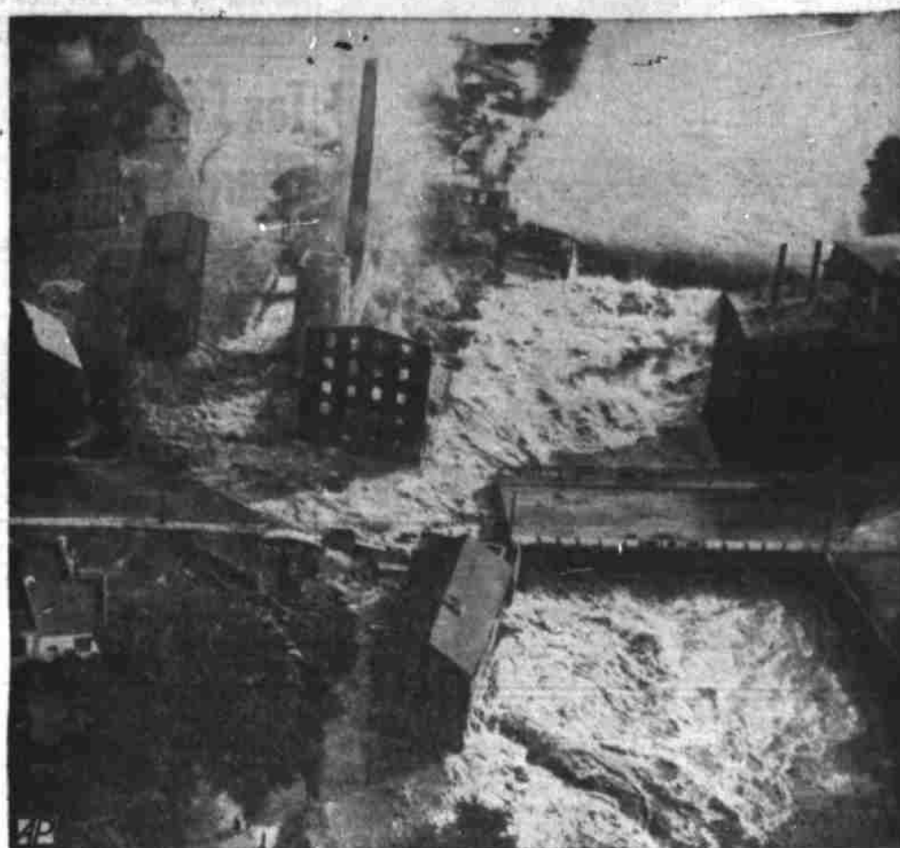
DOUBLE HAVOC — Flood waters of Quinebaug and French Rivers reached this magnesium plant's boilers at Putnam, Conn., last August, causing fire and preventing firemen from reaching scene. It was first of two New England floods which followed in the wake of hurricanes.
