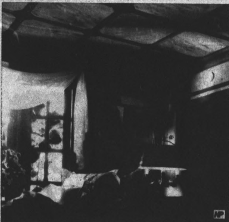
This suspended ceiling's faux marble finish is an example of what can be accomplished by customizing. In this case, fluted ceiling panels from Armstrong's Prestige Collection were marbled in a "Norwegian Rose" design to create a classic pavilion effect.
