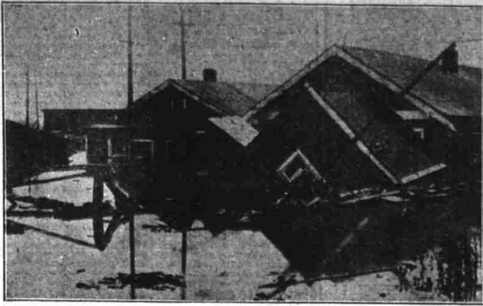
Waters from the swollen Puyallup river did extensive damage in lowlands near Tacoma, Wash., tearing out bridges, roads and railroad tracks and surrounding homes as shown here. (Associated Press Photo)
