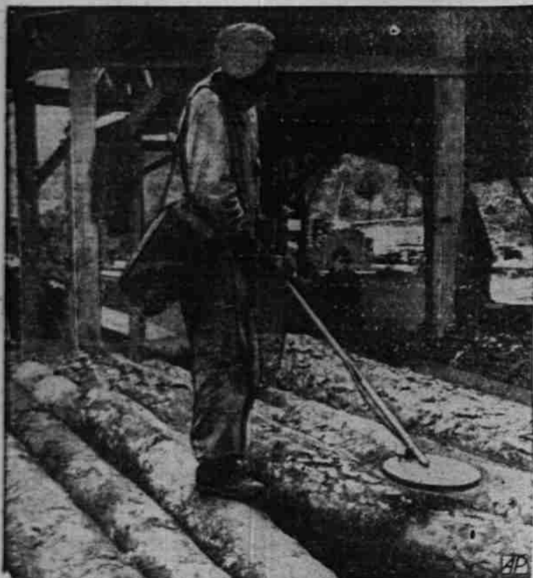
SAVING SAW BLADES —A POW at a saw mill in Grunewald forest, Germany, uses a mine detector to locate hidden fragments of bomb splinters before the logs are sawed.
