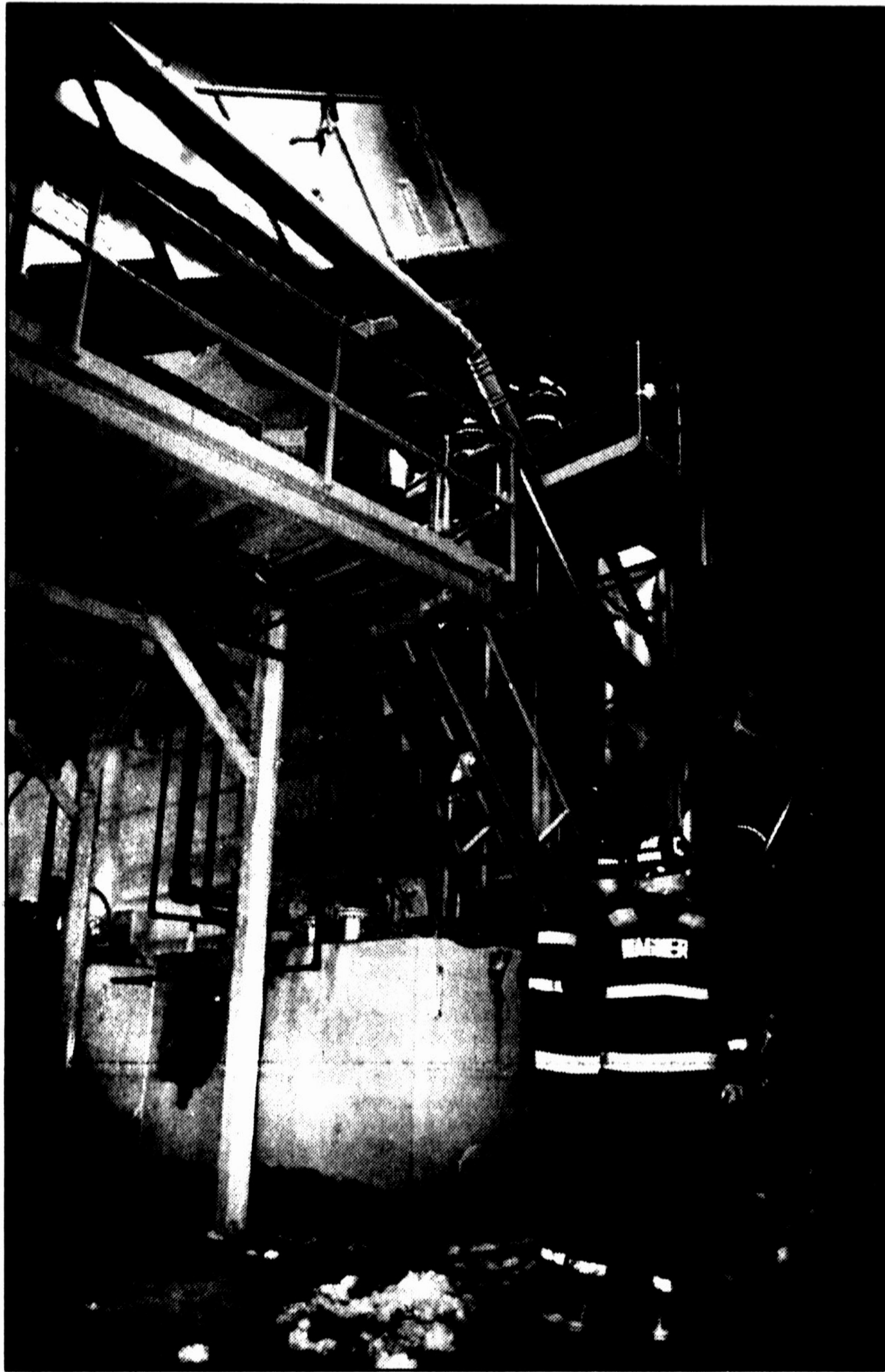
Hereford firefighters check damage to the Hereford Farmers Co-op gin following a fire Wednesday evening at the cotton-ginning plant located on South Main Street. Hereford Fire Marshal Jay Spain said this morning the fire apparently was ignited by a bolt that had worked loose and caused a spark. Spain said damage to the gin was minimal.
