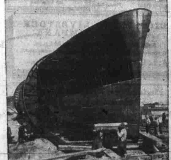
BOTTOMS DOWN —Upright, the subchaser being built by Defoe at Bay City, Mich., is ready for its prefabricated superstructure. These boats are for navy's inshore patrol. A launching table lowers the boat finally into the water.
