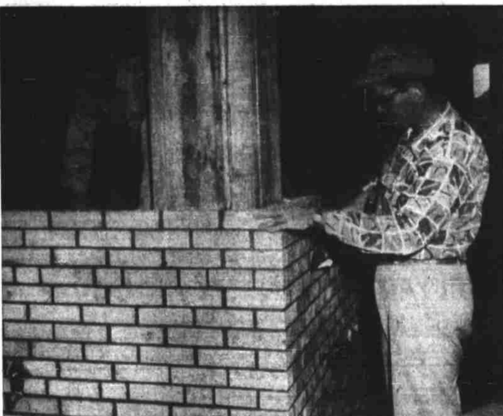
Brick Work Going Up
