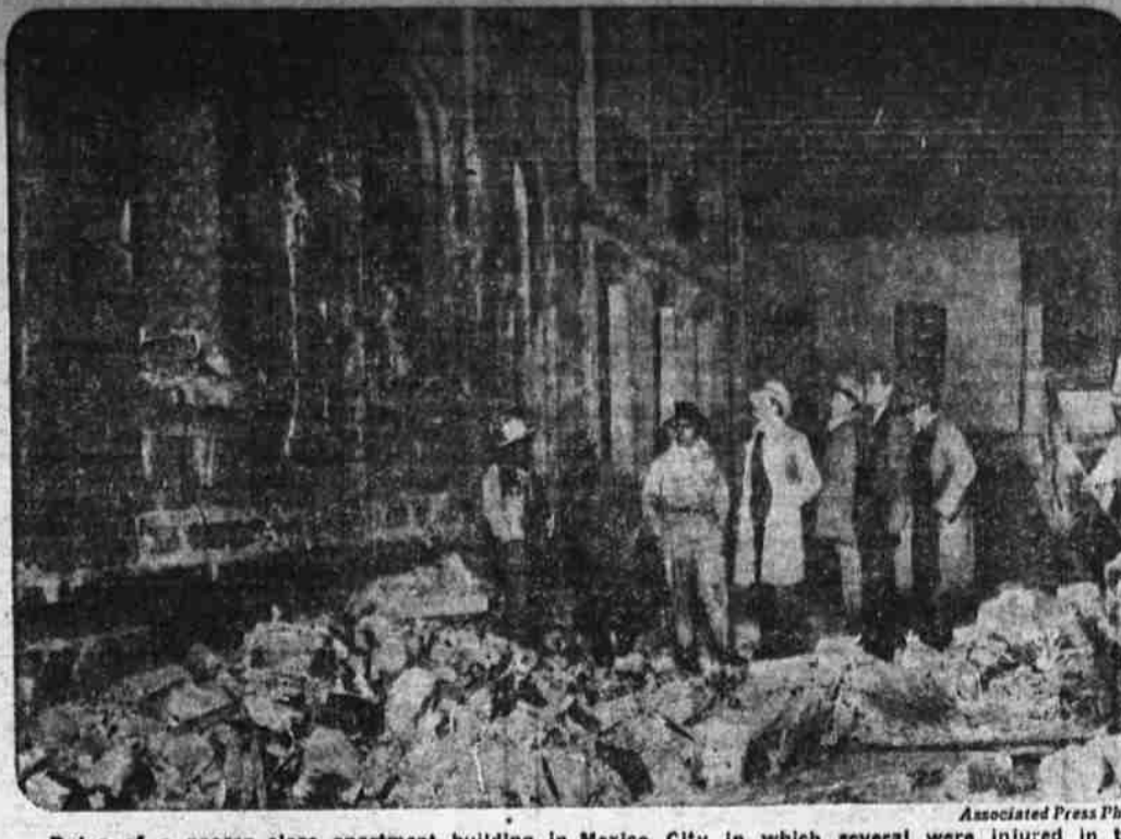
Associated Press Photo Ruins of a poorer class apartment building in Mexico City in which several were injured in the earthquake which shook a large section of the country.
