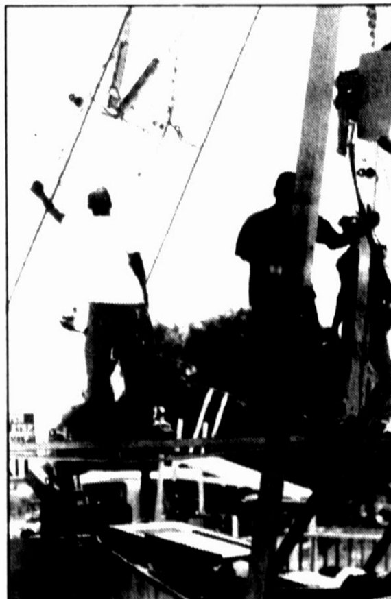
Assembling ferris wheel — Workers check the framework of the ferris wheel as they assemble the ride before the annual Lions Club Carnival, which gets under way at 7 p.m. today on the grounds of the Deaf Smith County Bull Barn. The carnival will be open 7-11 p.m. through Saturday and 6-10 p.m. Sunday.
