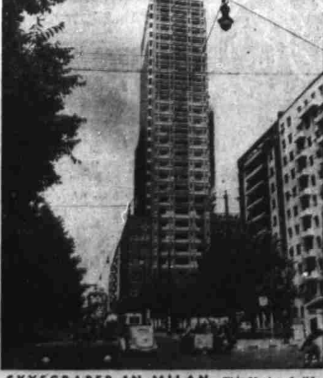
SKYSCRAPER IN MILAN — This 20-story building in Milan, Italy, is made entirely of concrete, including an atomic bomb shelter. Shops and offices occupy first nine stories and other 11 are devoted to private apartments.
