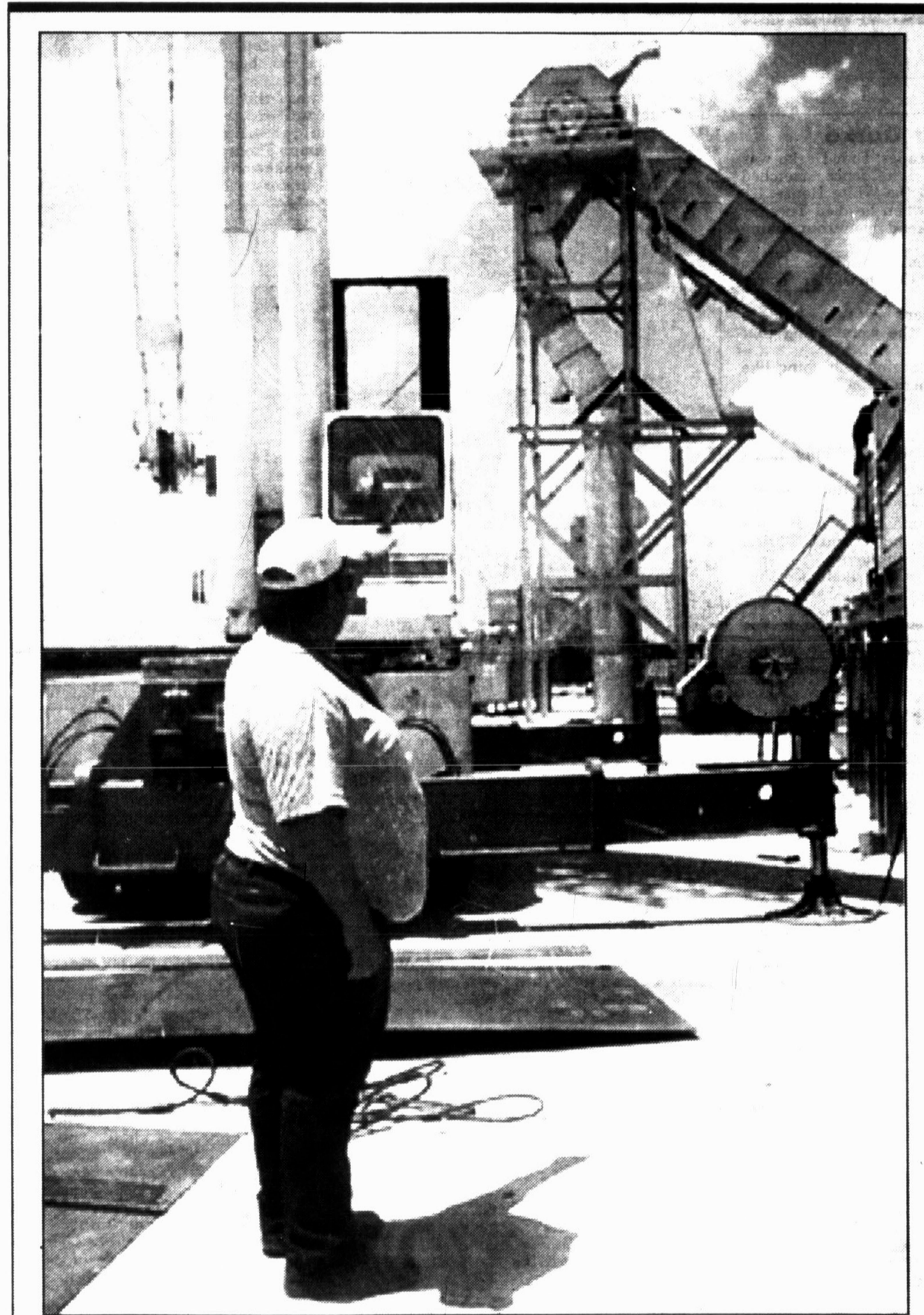
Cotton gin improvements — Hereford Farmers Co-op manager David Varner looks at the lint removal equipment installed Tuesday at the gin. The cooperative installed new equipment in preparation for the 1999 cotton harvest. The cooperative spent $1.5 million installing a single-stage saw lint cleaning process that replaces the old double process.
