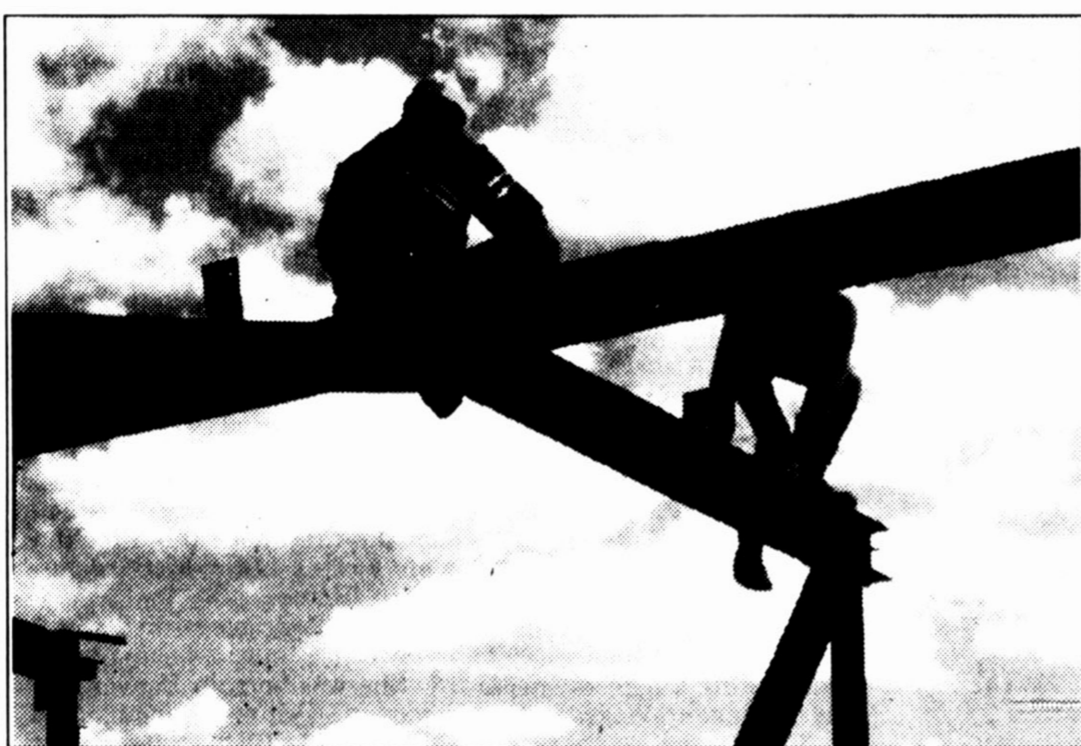
Two steelworkers erect the frame of new building at Hereford Junior High
