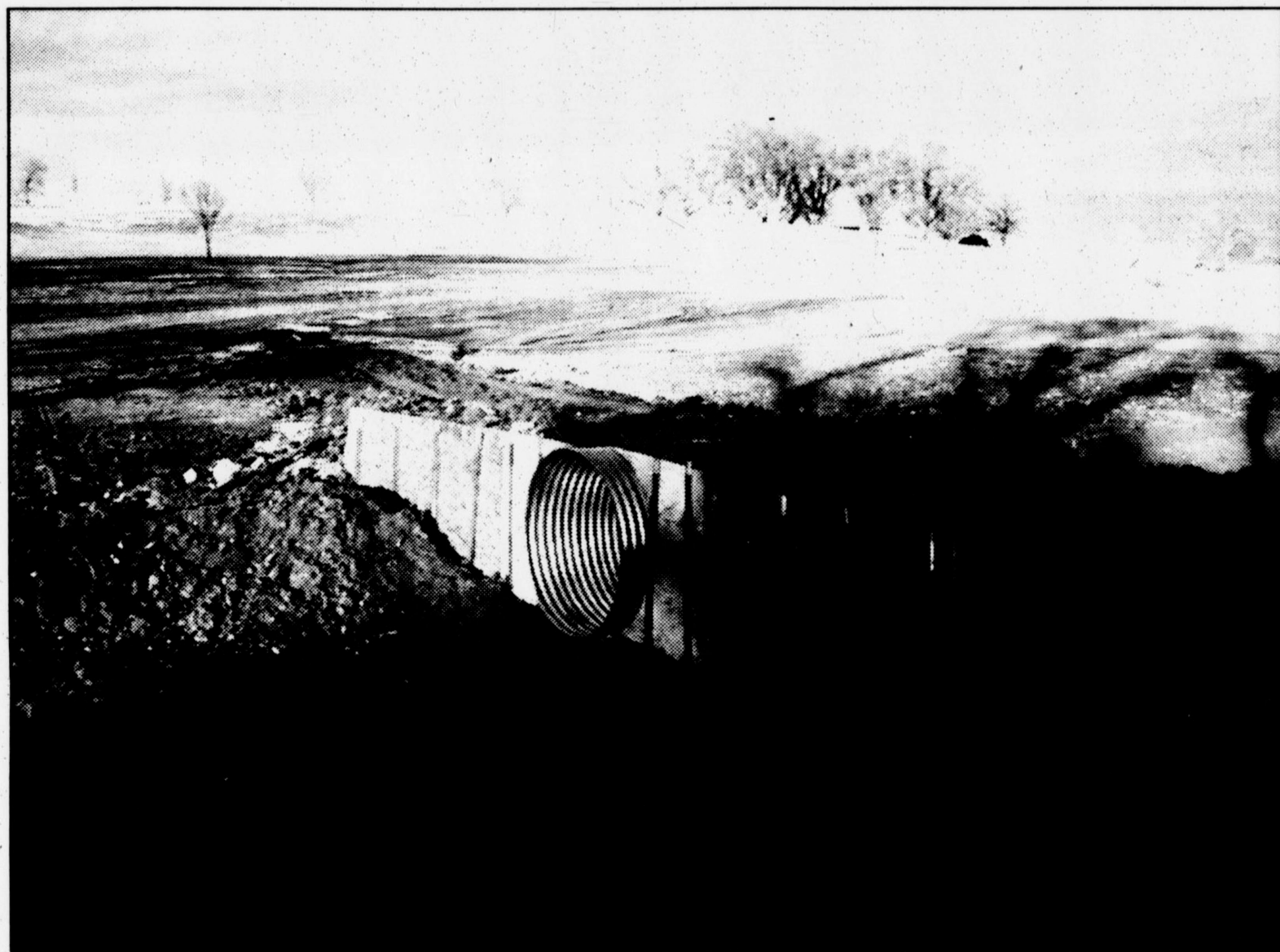
City of Hereford maintenance crews are installing a culvert between the 12th and 13th fairways at John Pitman Municipal Golf Course. Work continues at the course to repair damage caused by a flood in October 1998. Course superintendent Craig Nieman said a complete estimate is currently unavailable as the project is ongoing. He said about $10,000 has currently been spent in completing repairs to the course.
