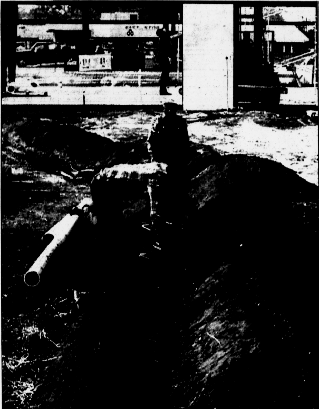
Laying line -- Henry Johnson (rear) and Joe Krck (correct spelling) of Henry's Plumbing lays a water line for Dean Crofford's automotive repair business, which is under construction in the 200 block of North 25 Mile Avenue.
