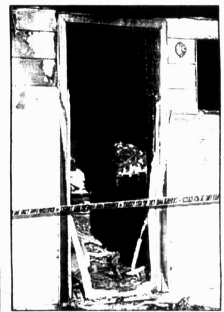
Photos by Mauri Montgomery
