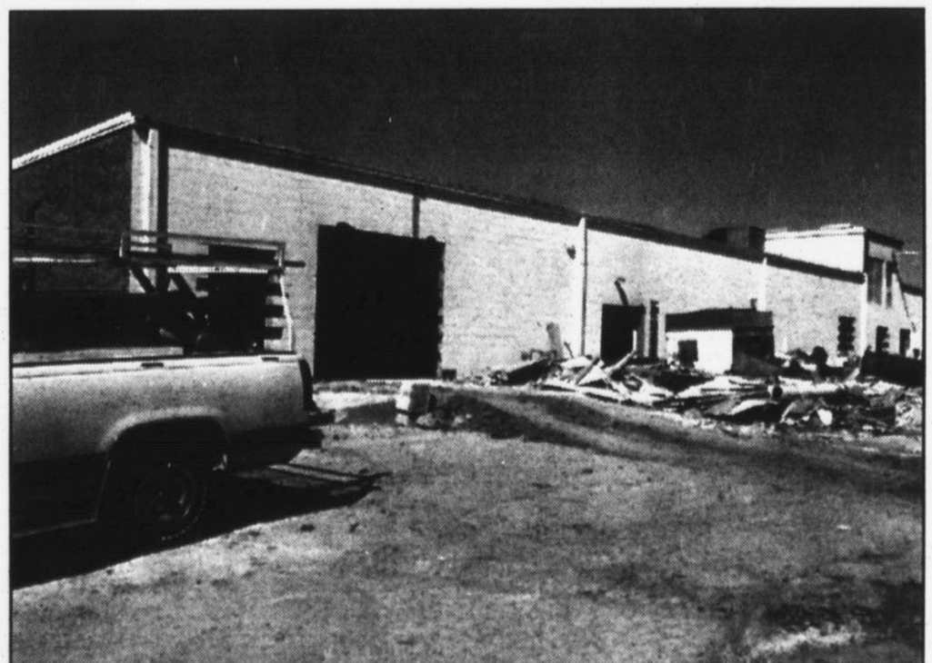
Construction on Moovies Six begins at Sugarland Mall
