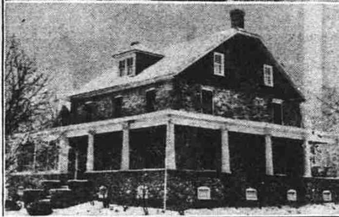
These houses, a far cry from the queenship of England for which she is now bidding, figured prominently in the early life of Mrs. Wallis Simpson for whose love King Edward was reported ready to abdicate his throne. Top, is shuttered and deserted clapboard residence in Blue Ridge Summit, Pa., where Mrs. Simpson was born in 1896. Below, summer cottage in same place where she lived with her mother as a girl of ten. Old time residents remember little of her. (Associated Press Photo)
