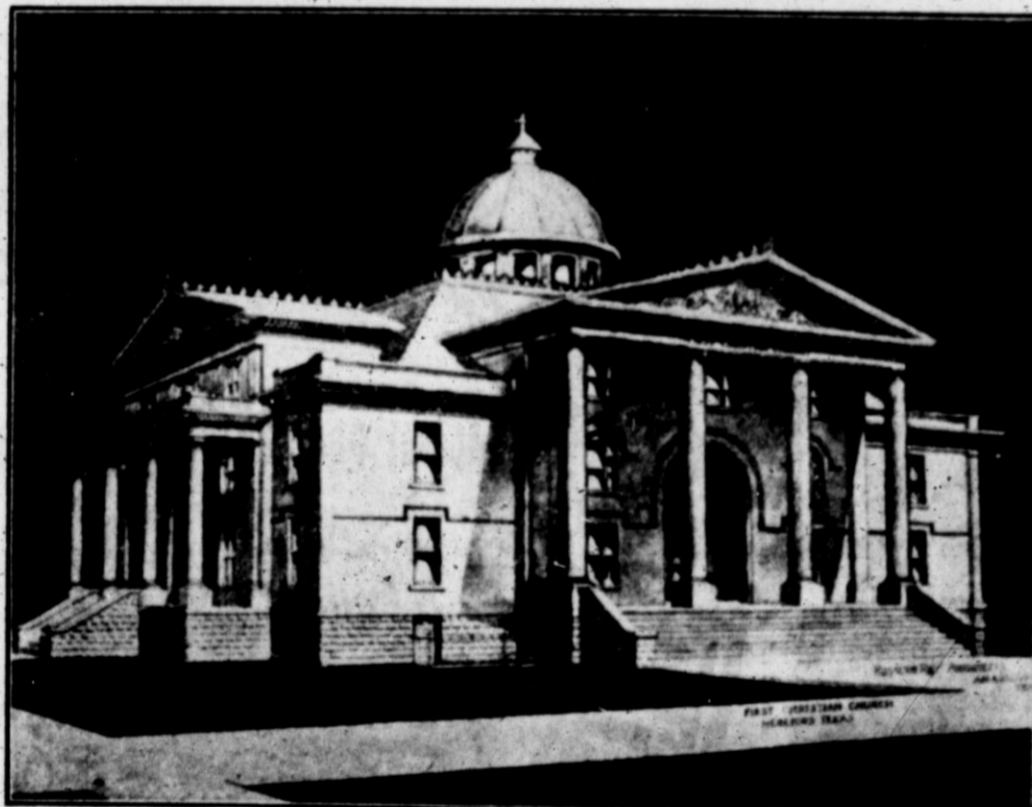
CONTRACTORS: Sam Worley and U. H. Kirby, foreman all woodwork and steel ceiling; Copes & Palmer, all roofing and sheet metal work. J. L. Johnson, all concrete block and cement work. T. L. Pearson, plumbing.
