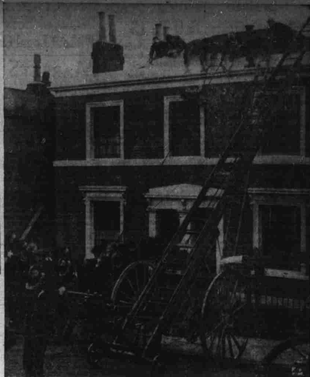
ROAMER ON THE ROOF-TOP brought London firemen hurriedly to the scene—a hour near the London county council Maudsley hospital. Only after a doctor ascended ladder would the girl, a hospital patient, agree to leave. Here she is being lowered to earth.
