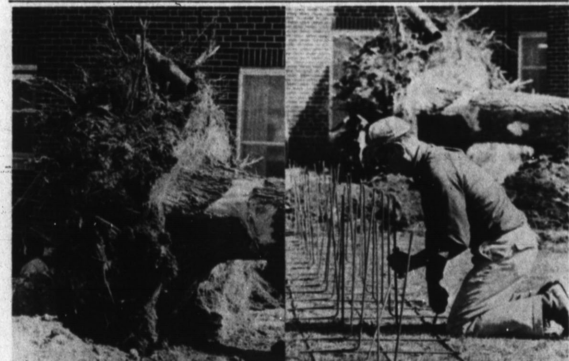
HOSPITAL CONSTRUCTION — Construction has begun at the Deaf Smith County Hospital to build a new room to house the new X-Ray equipment,
