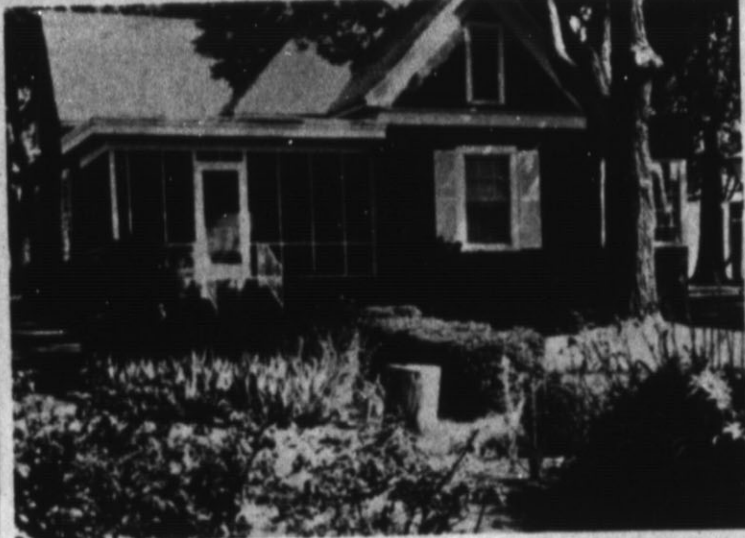
BUILT IN 1908 — From the front screened porch in the house the Coneways have lived in for 33 years, the two enjoy many hours of quiet, shattered only by cars traveling along South Main Street.
