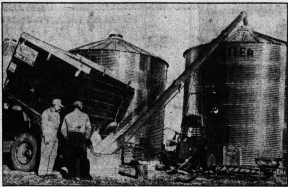
SAVING THE HARVEST —Farmers pour grain into one of the aluminum bins set up by the government at Enterprise, Iowa, to provide storage for the unexpectedly large 1949 grain harvest. About 26,000 bins were erected with an average capacity of 3250 bushels each to help meet the harvest emergency.
