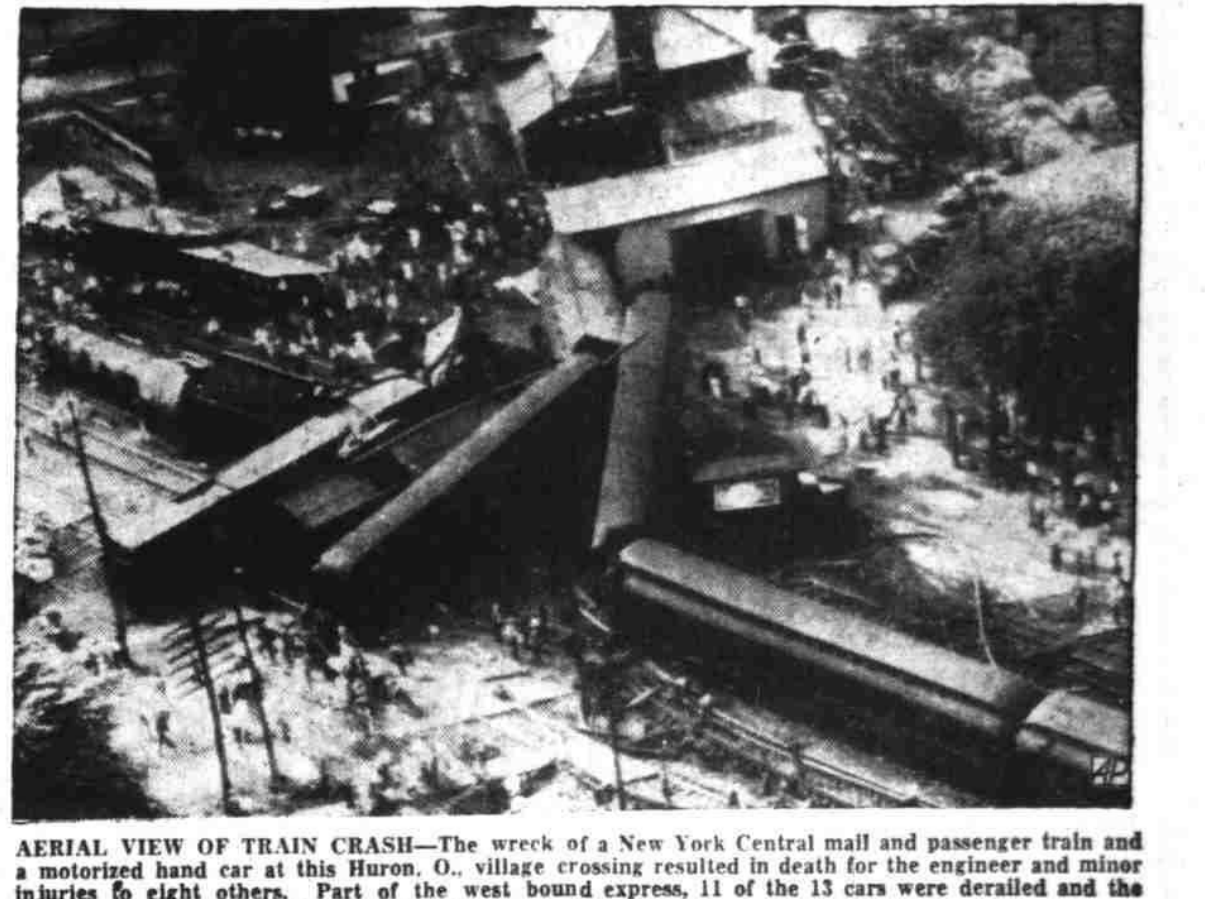
AERIAL VIEW OF TRAIN CRASH—The wreck of a New York Central mail and passenger train and a motorized hand car at this Huron, O., village crossing resulted in death for the engineer and minor injuries to eight others. Part of the west bound express, 11 of the 13 cars were derailed and the engine was overturned. (AP Wirephoto.)
