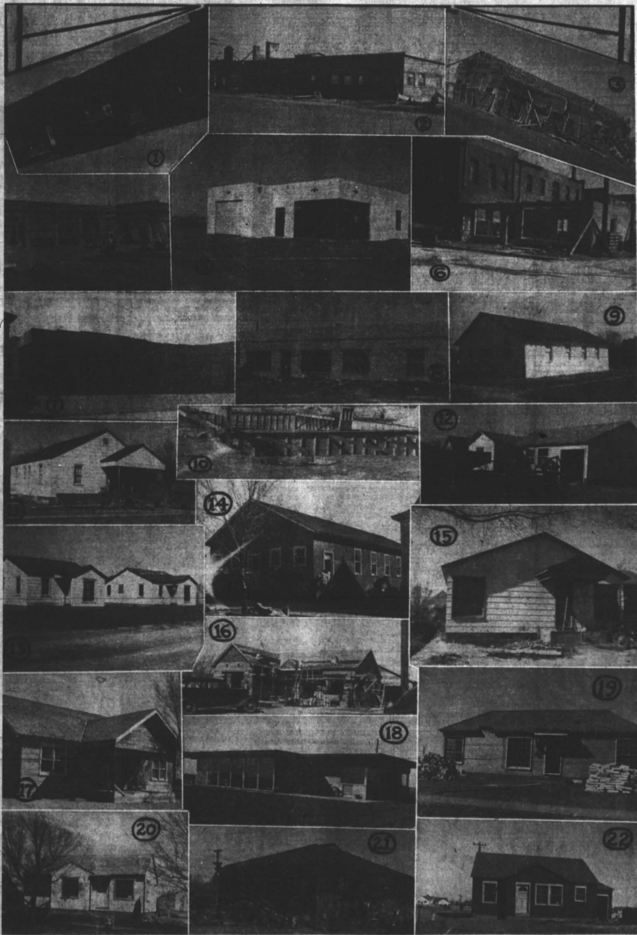
Here are few of the new houses and buildings now under construction in Hereford: (1) An addition to the Witherspoon building on East 2nd street; (2) the new Benefield Motor Company building on West 1st street; a garage and implement building under construction by Herschel E. Miller on East 1st street; (4) A filling station, cafe and grocery built by Roy Wagner on East 1st street; (5) A new filling station under construction east of town on Highway 60. (6) Addition to the Witherspoon building at rear of First State Bank. (7) new store buildings on Sampson street, one of which is already occupied by Western Battery and Electric; (8) Moore and Sowell Service Station at 1st and Kinney; (9) new Church of the Nazarene completed in February. (10) basement for the Fullwood building north of City Hall. (11) S. J. Barclay home on East 5th street. (12) Floyd McGee home on West 10th street; (13) two new homes built by C. H. Forson on Avenue E. (14) new Baptist Mission church on 25-mile Avenue. (15) A. B. Christian home at 508 Miles; (16) new home under construction by S. O. Wilson on West 6th street; (17) Patterson home on East 5th street; (18) George Heard home south of town. (19) Dr. L. B. (Bud) Barnett's new home on East 5th street. (20) Carl Luke home on Bradley street. (21) Glenn Oliver home on West 3rd street. (22) J. C. Hromas home on West 10th street.
