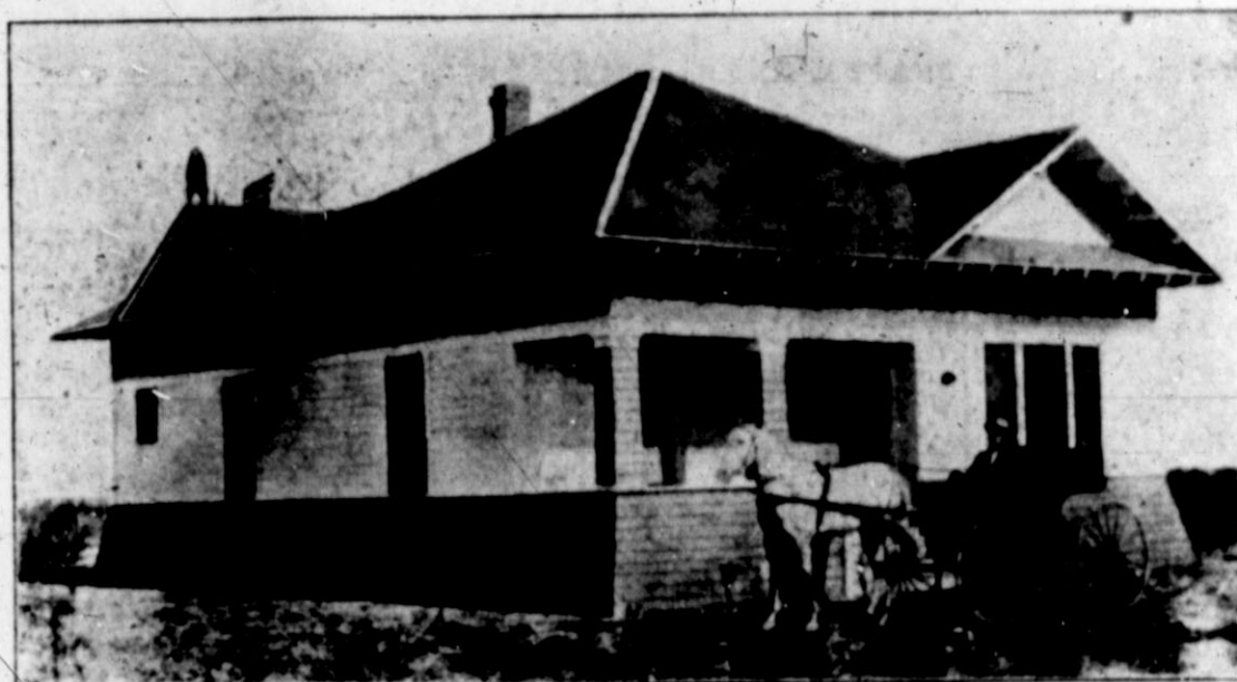
This is a Picture of the House We Give Away
