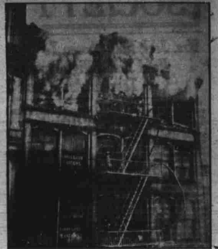
Employees of a paper-box factory on lower Broadway, New York City, were routed by flames and smoke when fire broke out in their building, but firemen (above) kept battling the blaze from fire escapes as it brought it under control. (Associated Press Photo)
