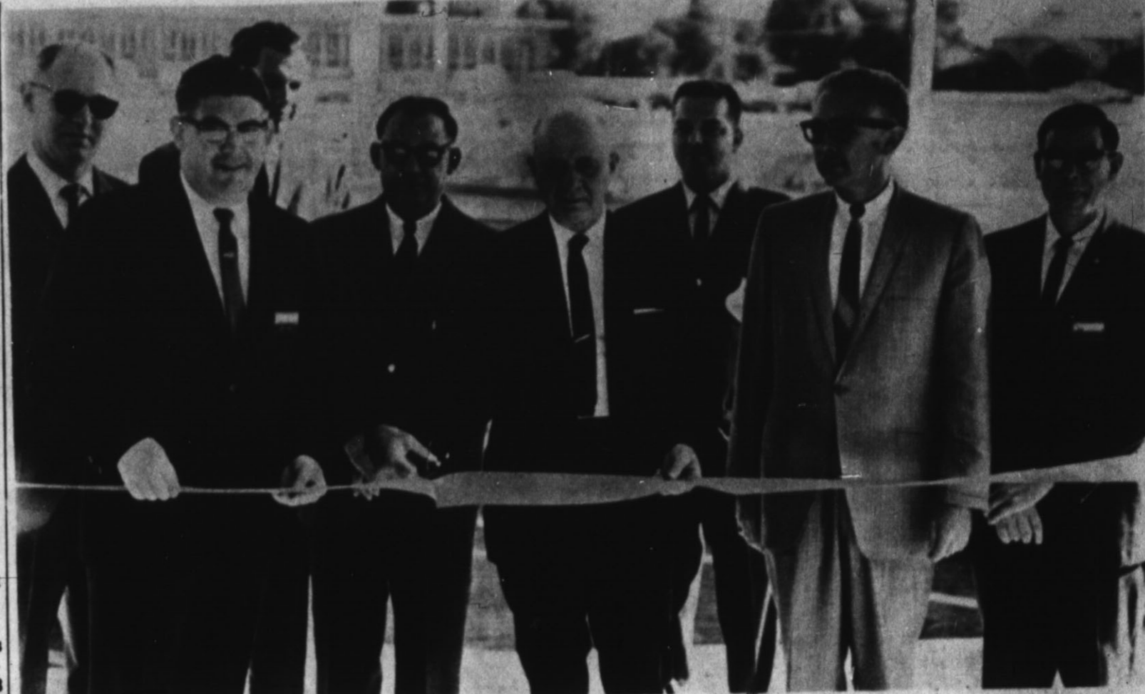
SAFeway OPENS — Hereford's Safeway store officially began business in their new Park Ave. Shopping Center store Monday morning at 7:45 with a ribbon cutting ceremony. Shown holding the ribbon at left is LeRoy McNally, Lubbock district manager of the chain store, while Mayor Ray Cowser cuts the ribbon. At right is Wayne Thomas,
