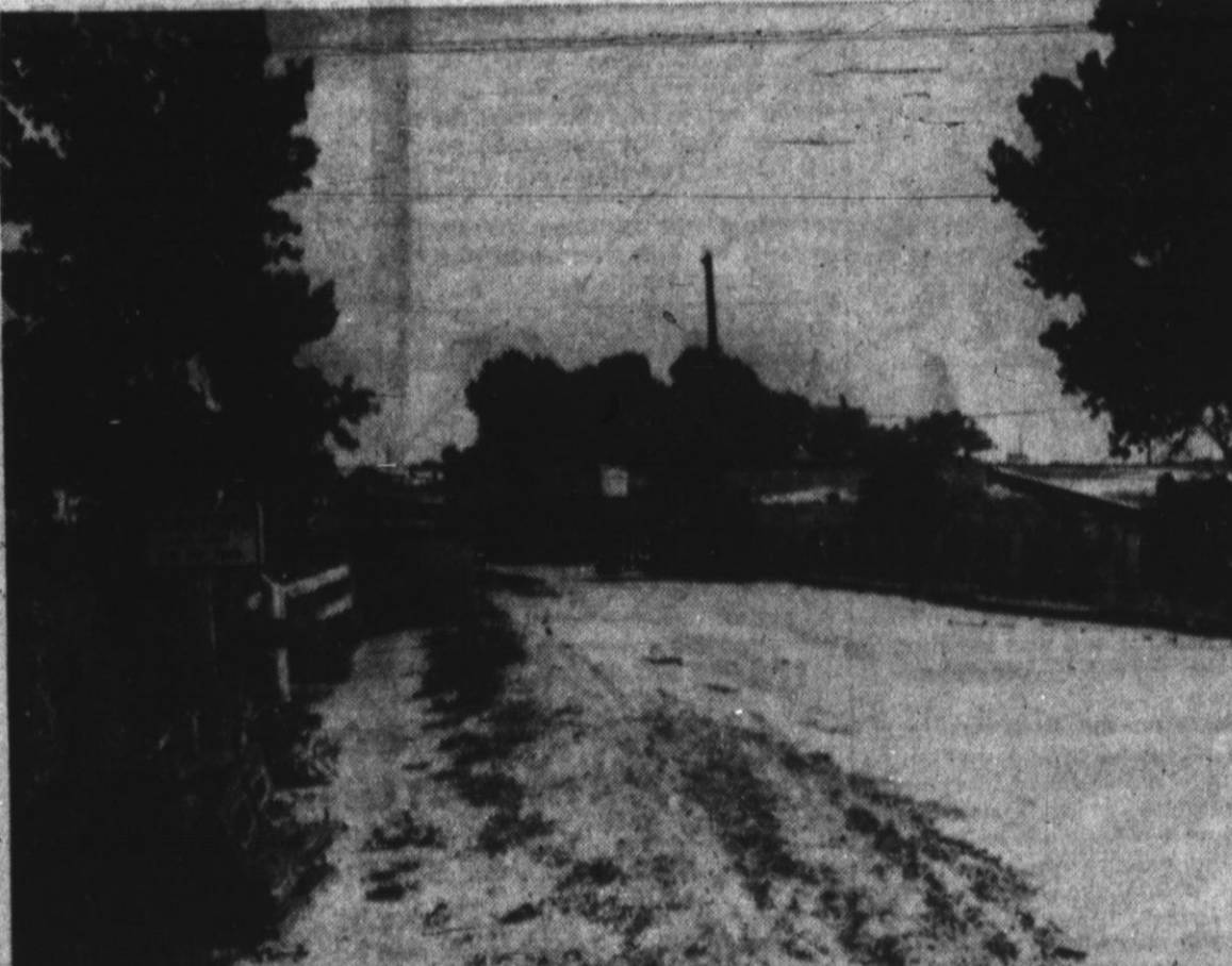
BRIDGE CONSTRUCTION on South Main just east of the city golf course, began this week. While the bridge is closed, through traffic will be detoured west to U. S. 385, according to W. Y. York, resident engineer of the state Highway Department. The bridge construction is one of the two projects started by the highway department in Deaf Smith County this week. (Staff Photo)
