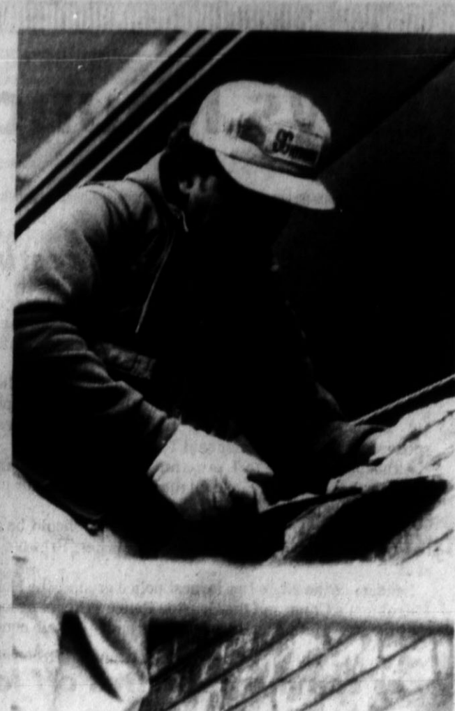
Step Four: Brick placement
