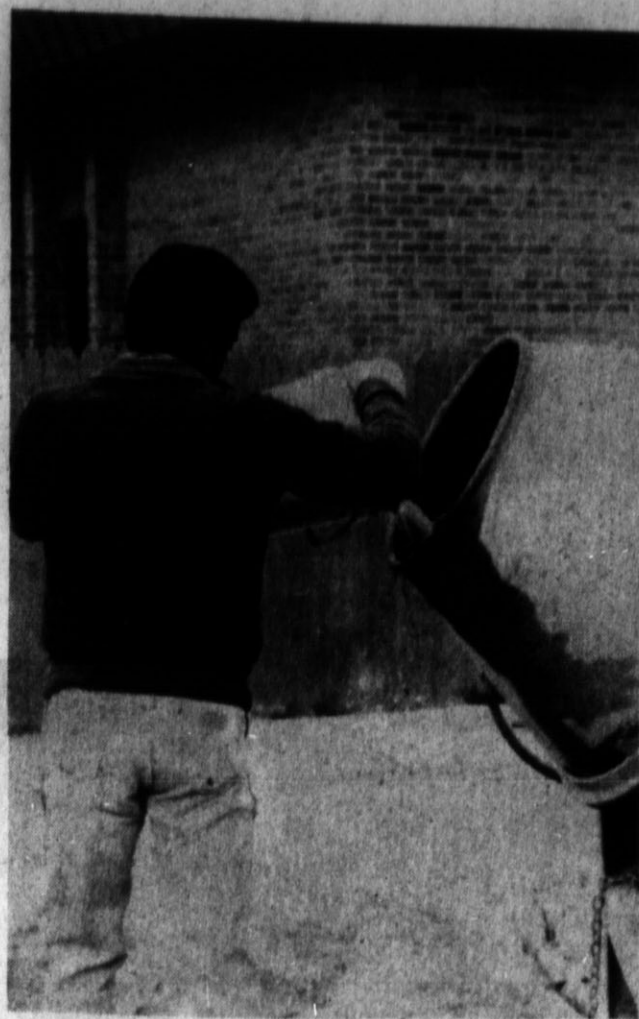
Step One: Mixing mortar
