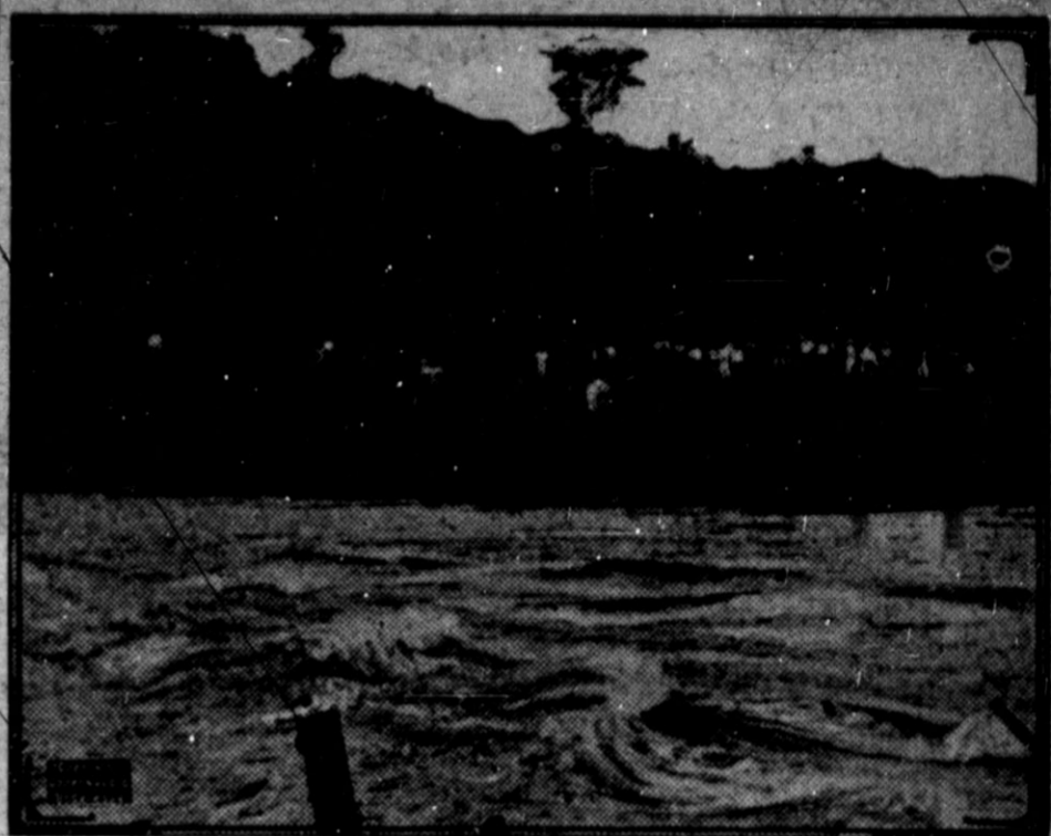
Like a mountain torrent the waters of Gatun Lake poured into Culebra Cut through the sixty-foot gap in Gamboa Dike made by the explosion of 1,600 pounds of dynamite. At Gold Hill the flood was partially dammed by the Cucaracha slide and within an hour and a half the cut was filled to lake level.
